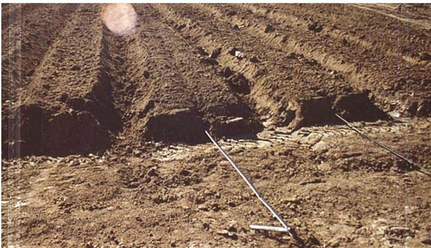
Drip tube connections should be perfect. Risers from pipelines should be accurately drilled. Extreme care is needed filling trenches. The system should be pressurised and loose fill delicately pushed into trenches to prevent movement and kinking of risers or tube.
